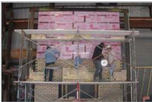
Figure 3: Test wall under construction
