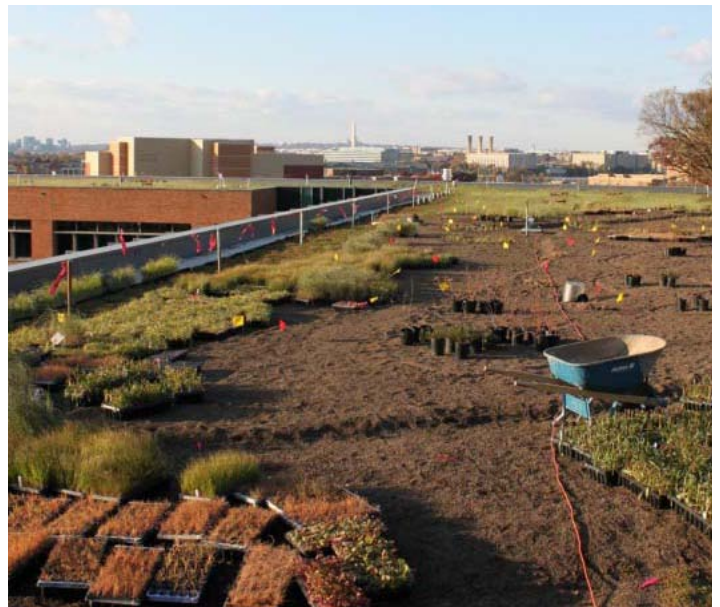
Sedum mats on the roof perimeter.
