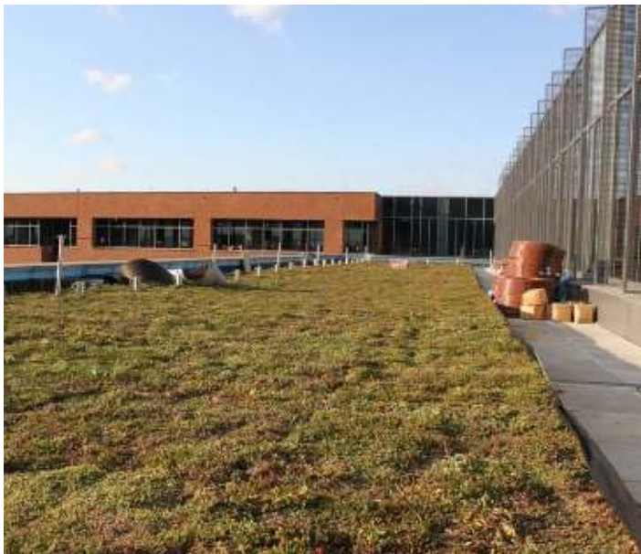
Roof planted exclusively with pre-grown sedum mats.
