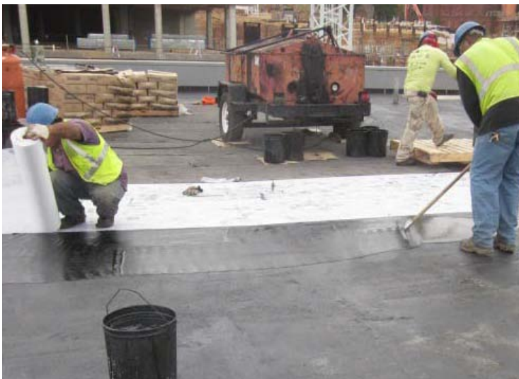
Crews installing hot rubberized asphalt.
